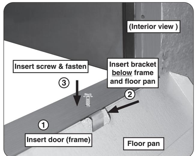
**Fig. 10-3** Door/floor pan install detail
