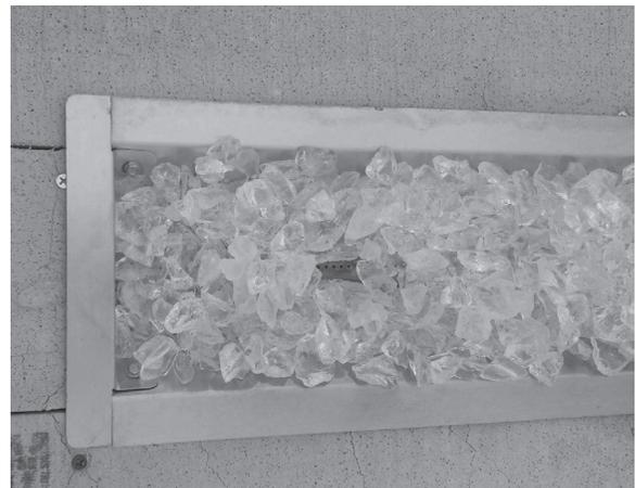
Figure 5.3 Pan Installed on Top of Finish Material
